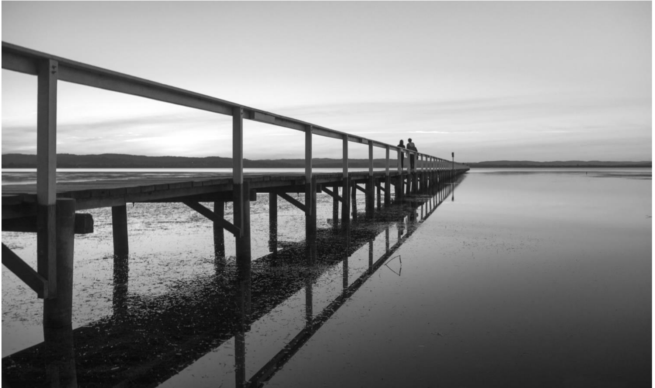
Long Jetty Chris Latham Credit
