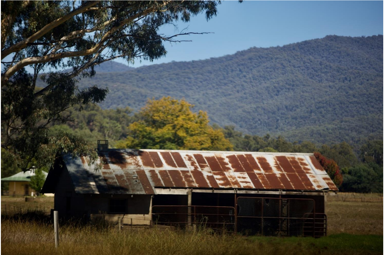
Rusty old Shed
